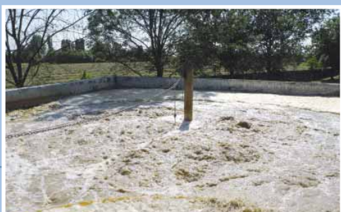
Aeratori sommersi tipo SC installati in impianto di depurazione. Submersible aerators type SC installed in a wastewater treatment plant.
